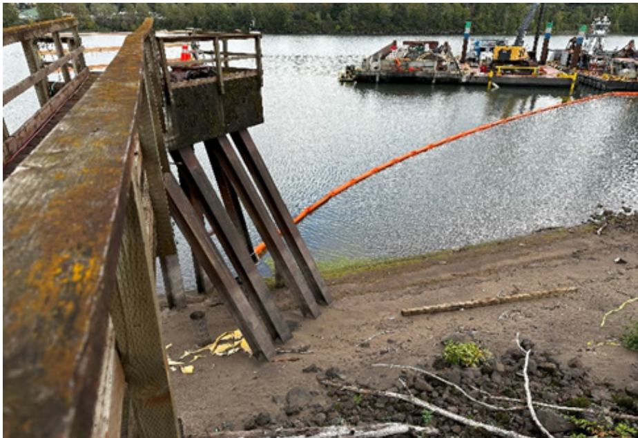
Downriver portion of replaced containment boom at sheen management area (10/25/2023).
