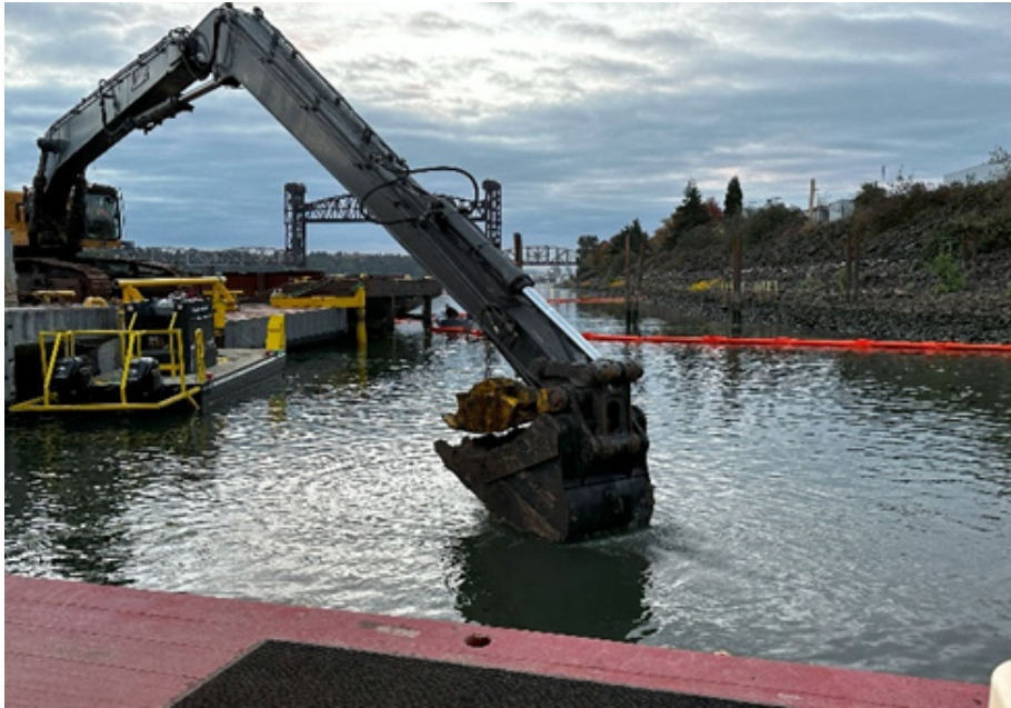
Placing sand in removed dolphin footprint (10/24/2023).
