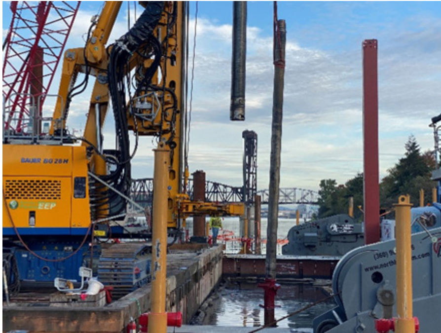
Attaching 3-foot auger bit to Bauer 28H drill rig (10/17/2023).
