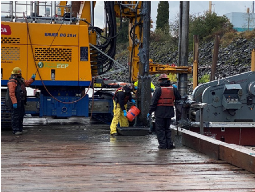
Collecting ISS QA/QC sample from middle interval of column 3-11 (10/16/2023).
