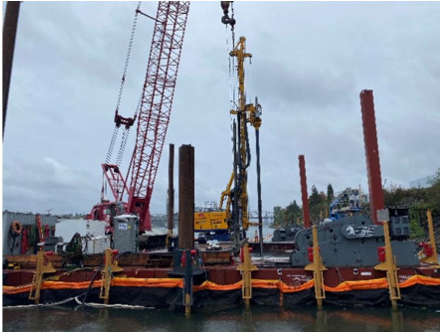
Performing ISS auguring at column 3-11 to 30 feet below mudline (10/16/2023).
