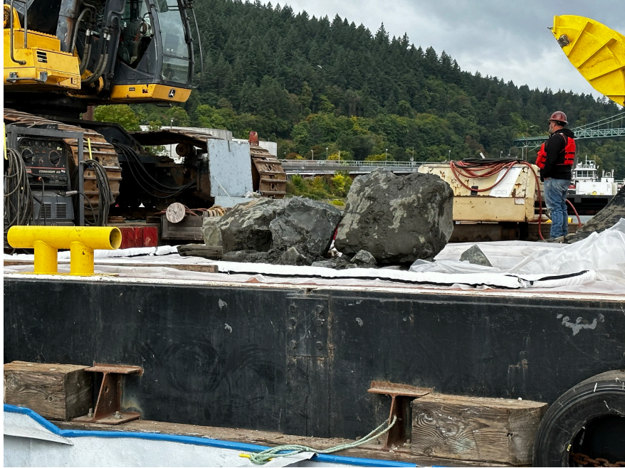
Removed debris placed on barge (9/20/2023). No sediment removed during debris removal operations.
