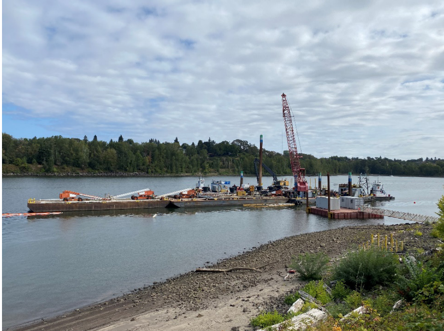
ISS barge and crane assembly with installed gangway to riverbank (9/18/2023).
