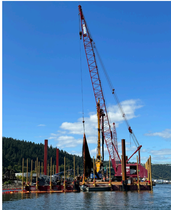
Silt curtain installation on ISS barge moon pool (9/19/2023).
