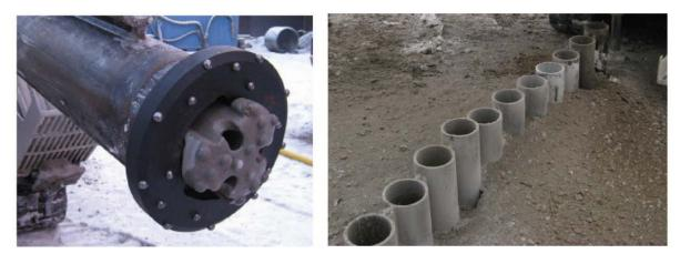
Exhibit Alt 2D-6: RD pile bit and downhole hammer (left) and view of top of piles after installation (right) (Uotinen and Jokiniemi, 2012)
