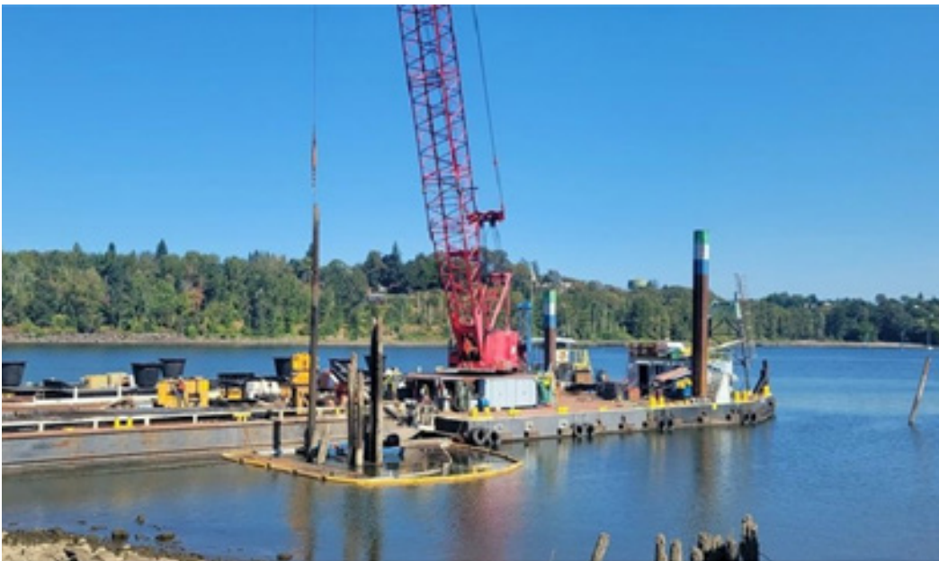
Extraction of pilings associated with former timber dolphin (9/15/2023).
