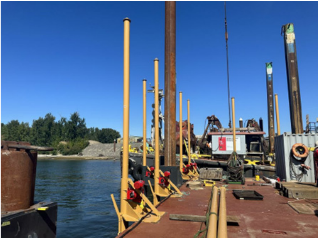
Installation of spuds and generators for ISS barge moonpool (9/13/2023).
