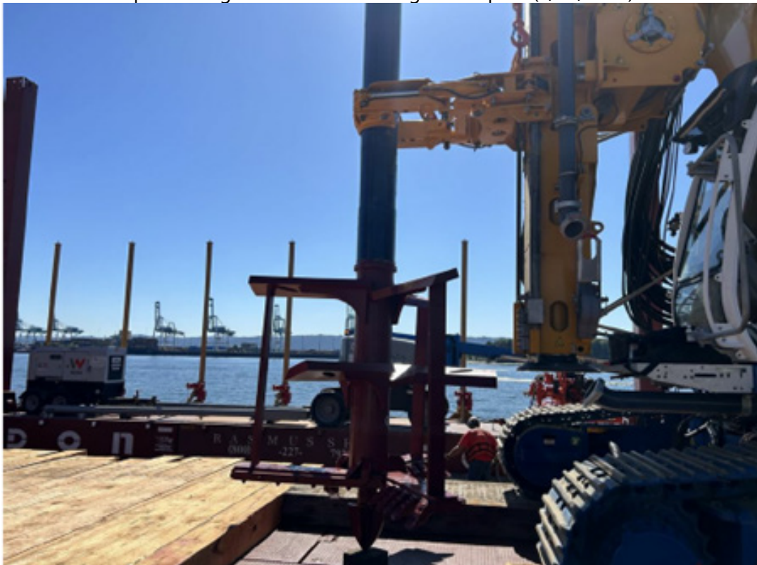
Mobilized Bauer 28 H drill rig (9/14/2023).
