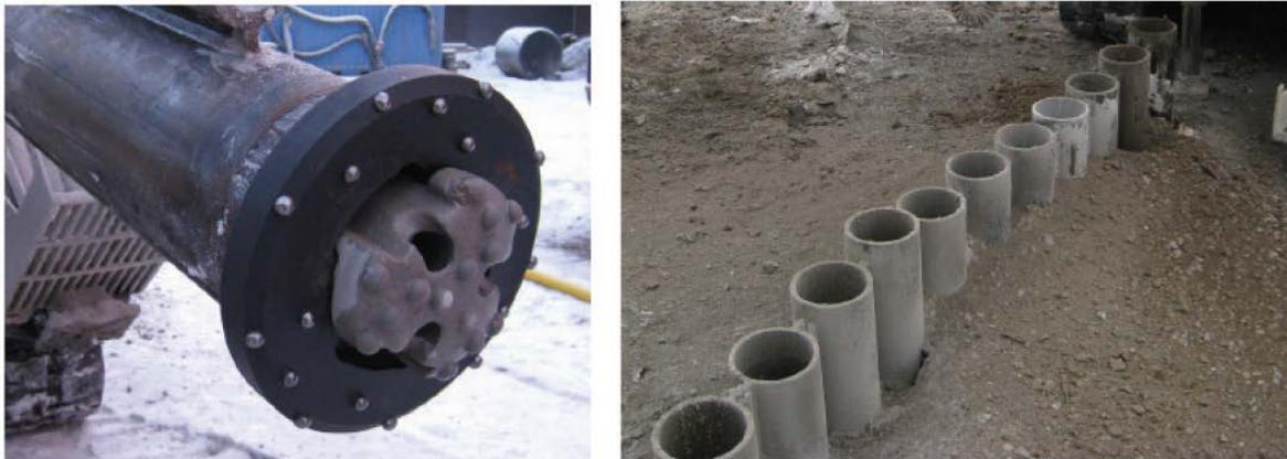
**Exhibit Alt 2D-6: RD pile bit and downhole hammer (left) and view of top of piles after installation (right) (Uotinen and Jokiniemi, 2012)**
