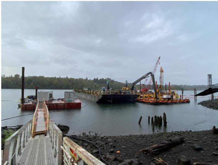
Excavator on swell material barge removing debris near column 4-1 (10/11/2023).
