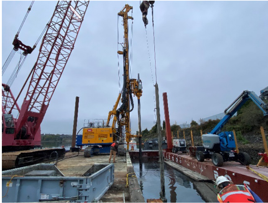
Performing ISS auguring at column 7-9 (10/04/2023).
