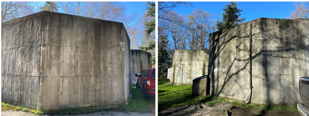
(L) & (R) Existing reservoirs – soon to be demolished once the new tank is finished and online
