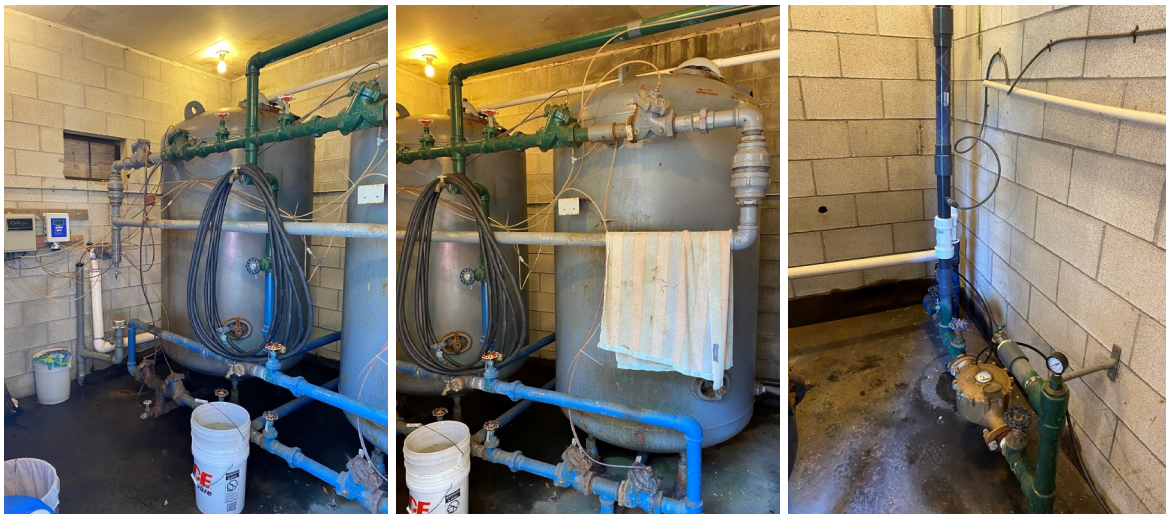
(L) & (Center) 2 filters at Island View site (R) Potassium permanganate injection point
