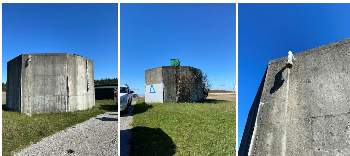
(L)Fort Nugent Reservoir (Center) For Nugent Reservoir (R) Screened overflow at Fort Nugent reservoir
