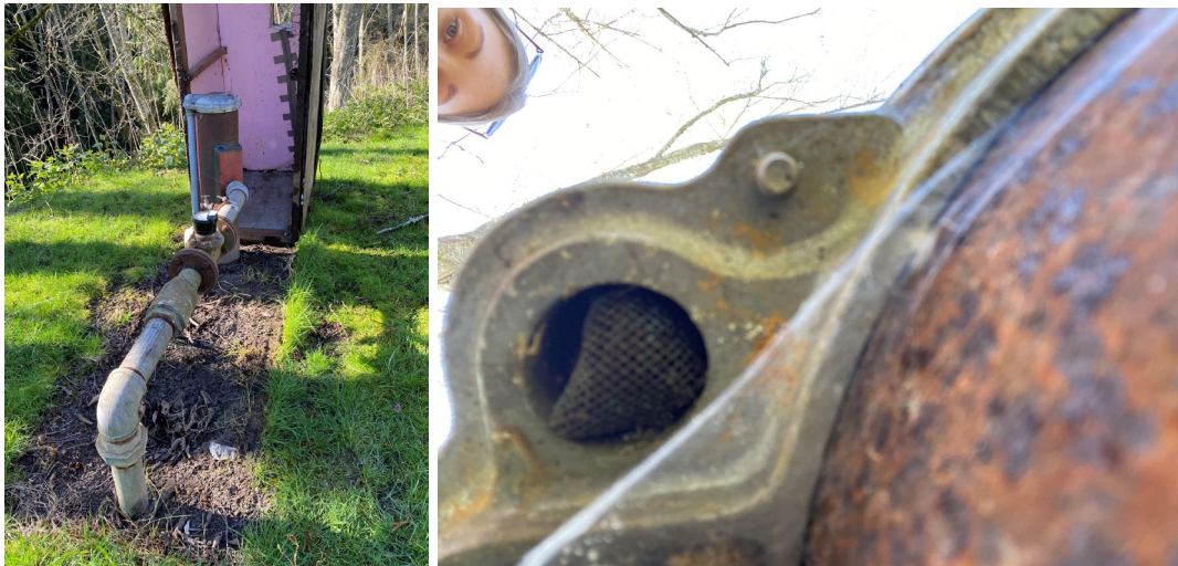
(L) Well #4 (R) Screened vent on Well #4 – screen bubbled but fully intact
