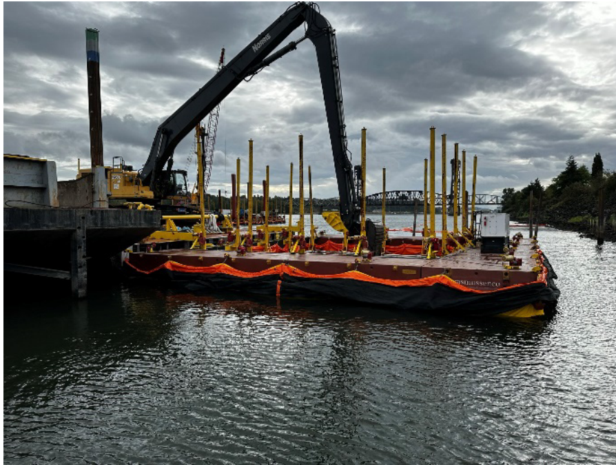
Performing debris removal at ISS column 1-4 (09/26/2023).
