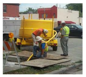
use of horizontal drilling accounted for as much as 83% to 95% of the pipe replaced. The illustration at right shows new main pipe being installed in the bore created by horizontal drilling.
