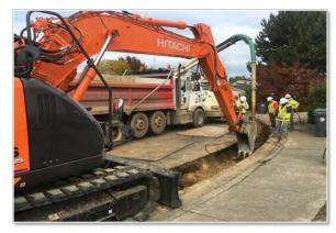
in established municipal areas and neighborhoods with existing paved roadways, sidewalks, landscaping, and other underground facilities. The illustration at left shows the pavement cut required for open trench installation of new main pipe.
