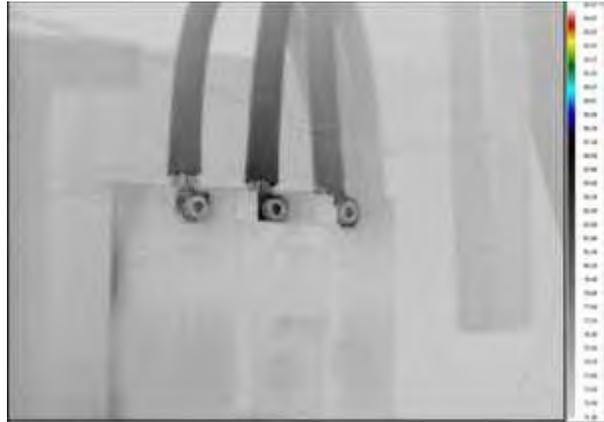
Simple repairs, such as cleaning and tightening connections, reduce the risk of equipment failure.
