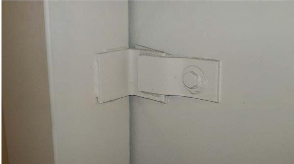
Photo 12: Concrete Wall to Column Clip
