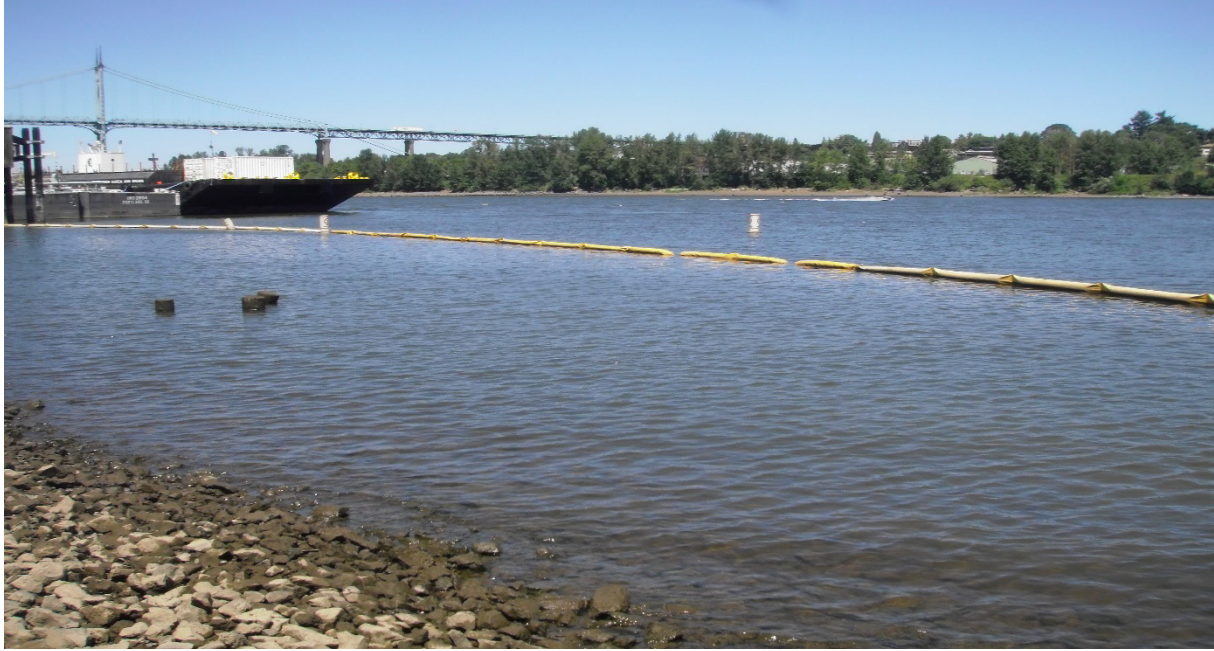
Photo 1 Centerline Logistics Oil Boom Placement from Dock to Dolphin with Three Mariner Warning Buoys at Pilot Cap Area (7/18/2023)
