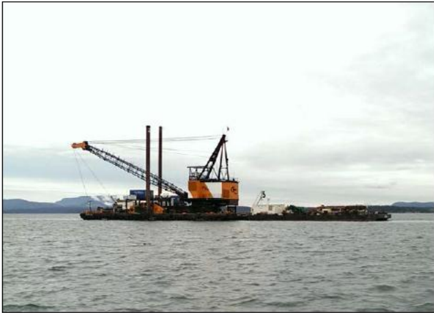
Figure 7 - Cable Repair Barge
