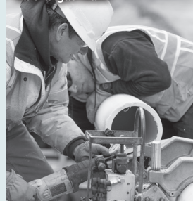
Crews install an upgraded natural gas main.
