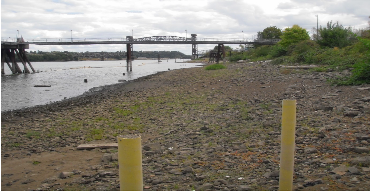
Photo 3 Conditions Immediately Downriver of Cap Area Looking Upriver Toward Cap Area (8/22/2023)
