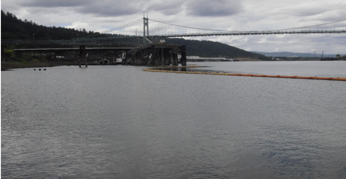
Photo 1 Centerline Logistics Oil Boom Placement from Dock to Dolphin with Three Mariner Warning Buoys at Pilot Cap Area (8/22/2023)
