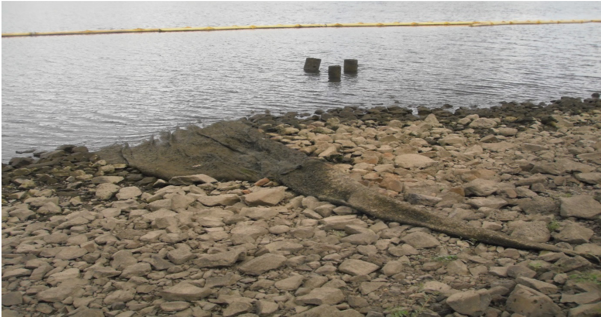
Photo 2 Organoclay Mat Material at the Upriver Extent of the Pilot Cap Area (8/22/2023)
