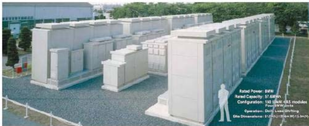
Figure 12- NGK NAS 8 MW (Japan)
