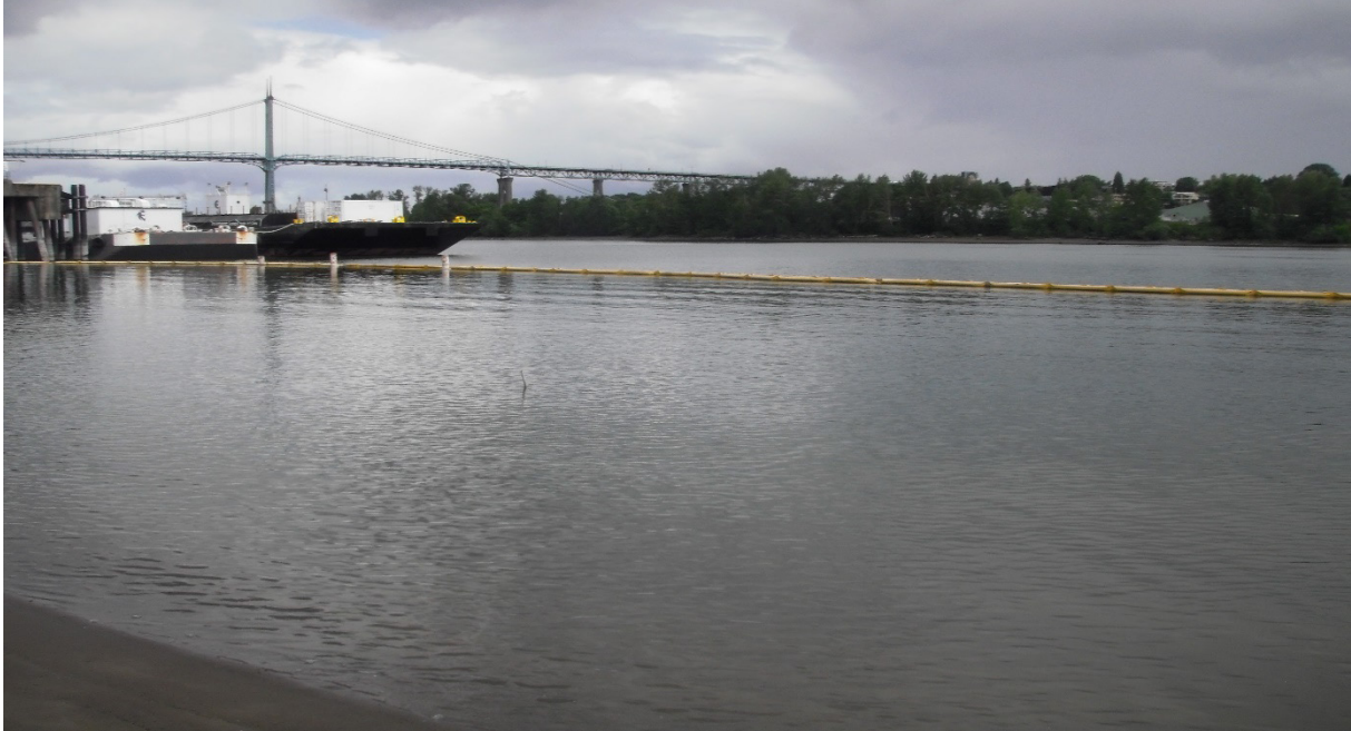
Photo 1 Centerline Logistics Oil Boom Placement from Dock to Dolphin with Three Mariner Warning Buoys at Pilot Cap Area (6/19/2023)
