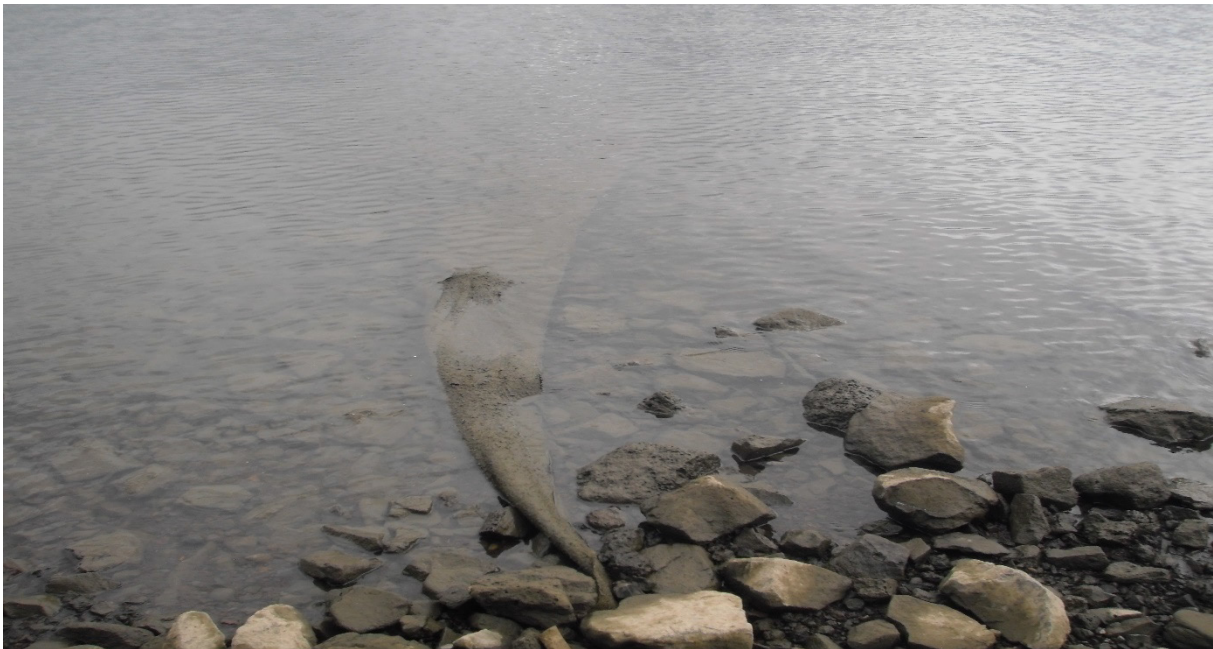
Photo 2 Organoclay Mat Material at the Upriver End of the Cap Area (6/19/2023)
