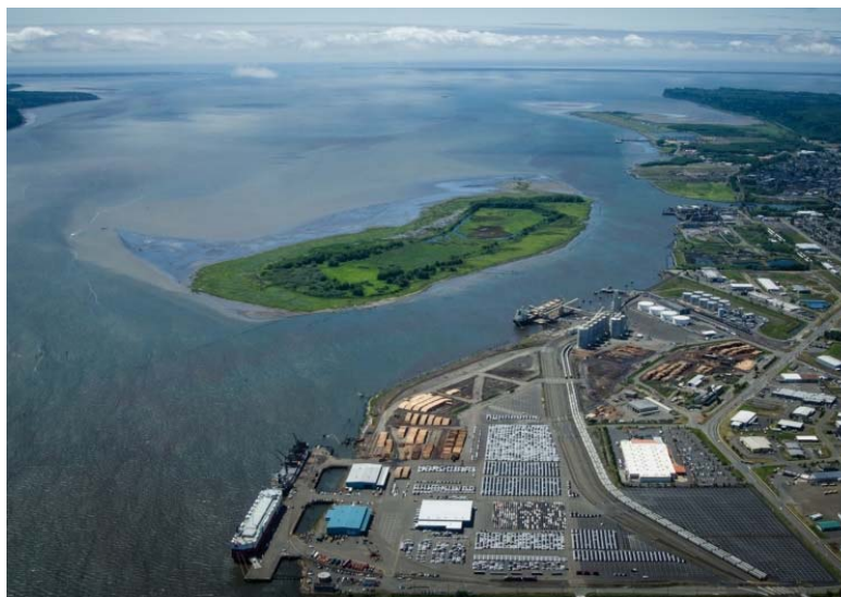
Aerial of the Port of Grays Harbor Operations. Photo courtesy of KBKW.
