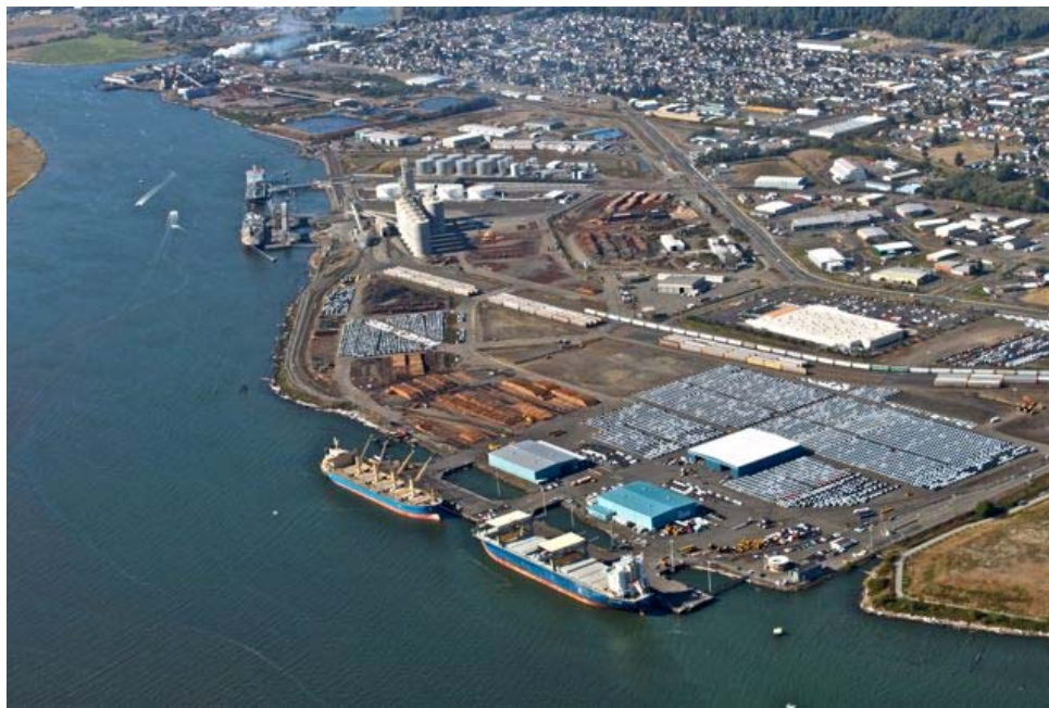
Aerial of the Port of Grays Harbor Marine Terminals. Photo Credit: Grays Harbor Talk
