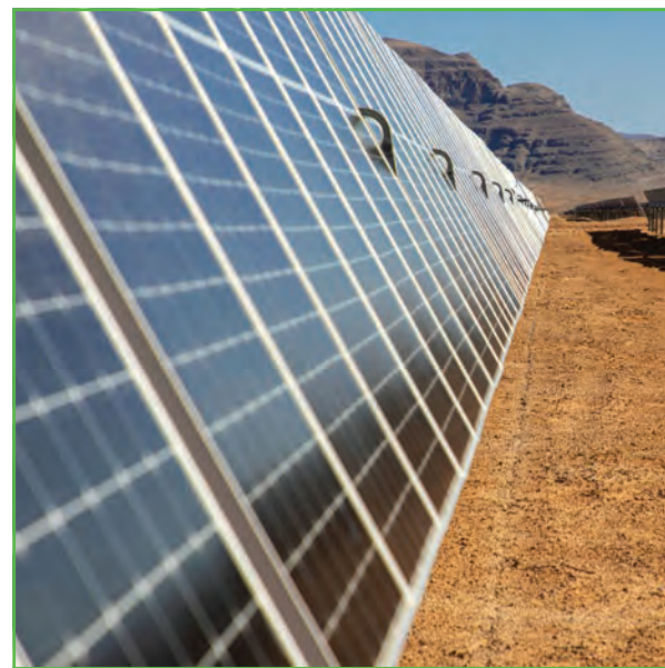
MDU Construction Services Group subsidiary Bombard Renewable Energy finished construction on a 200-megawatt solar facility in Nevada.
