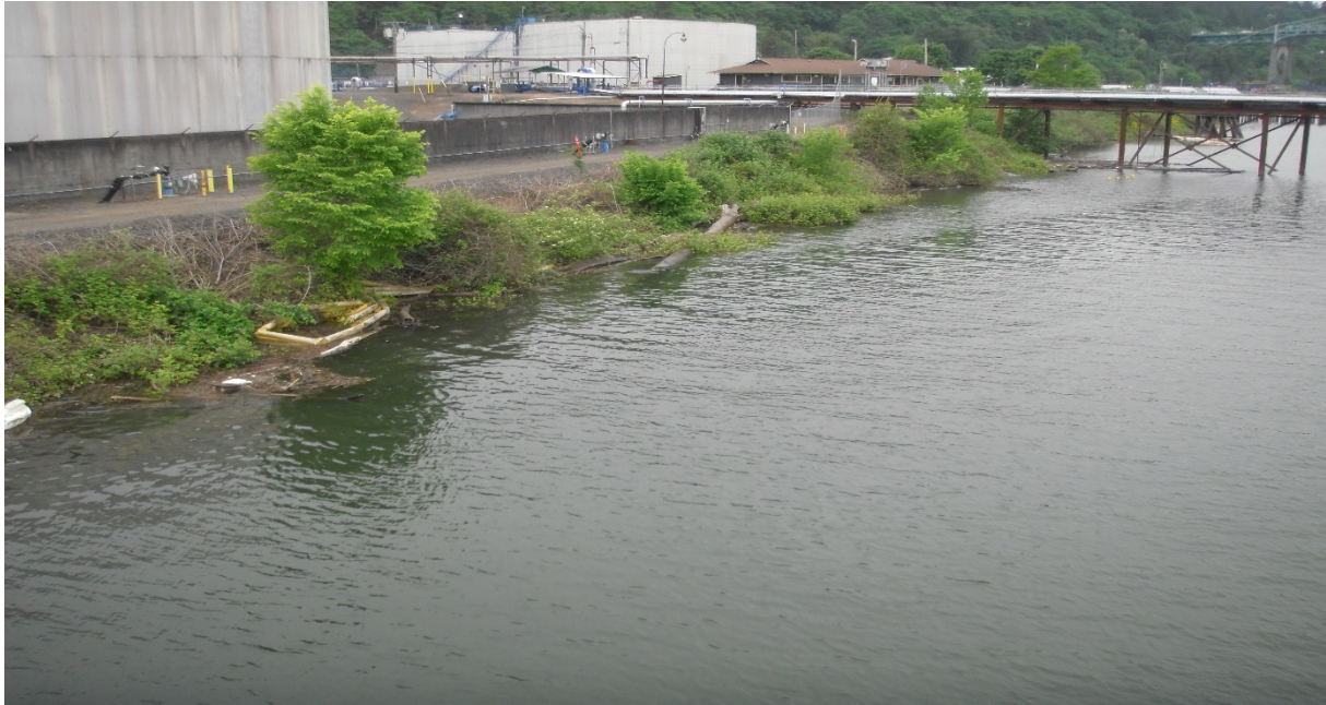
Photo 3 Conditions Immediately Downriver of Cap Area Looking from the Dock (5/19/2023)
