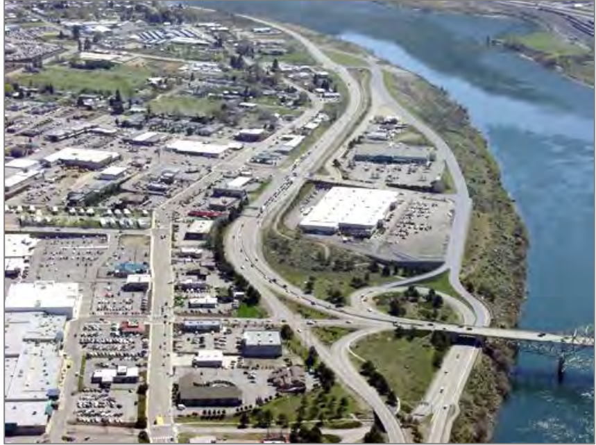
WSDOT recently completed modifications at the interchange of SR 28 with SR 285 including a southbound by-pass of the Grant Avenue intersection.
