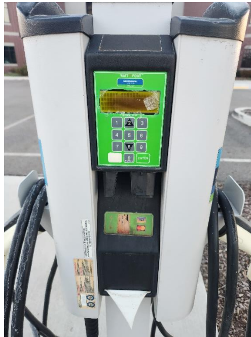
Figure 19: Payment module screen damaged and protective covering smashed.
