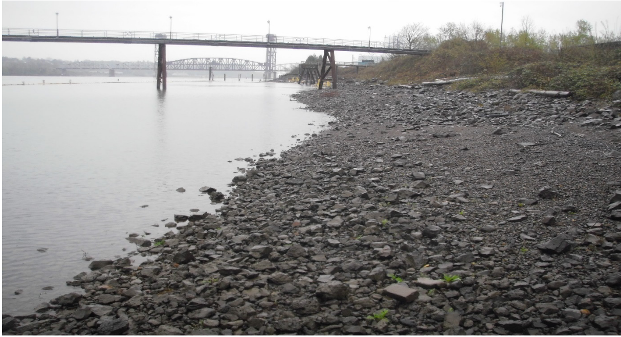
Photo 3 Conditions Immediately Downriver of Cap Area Looking Upriver (4/20/2023)
