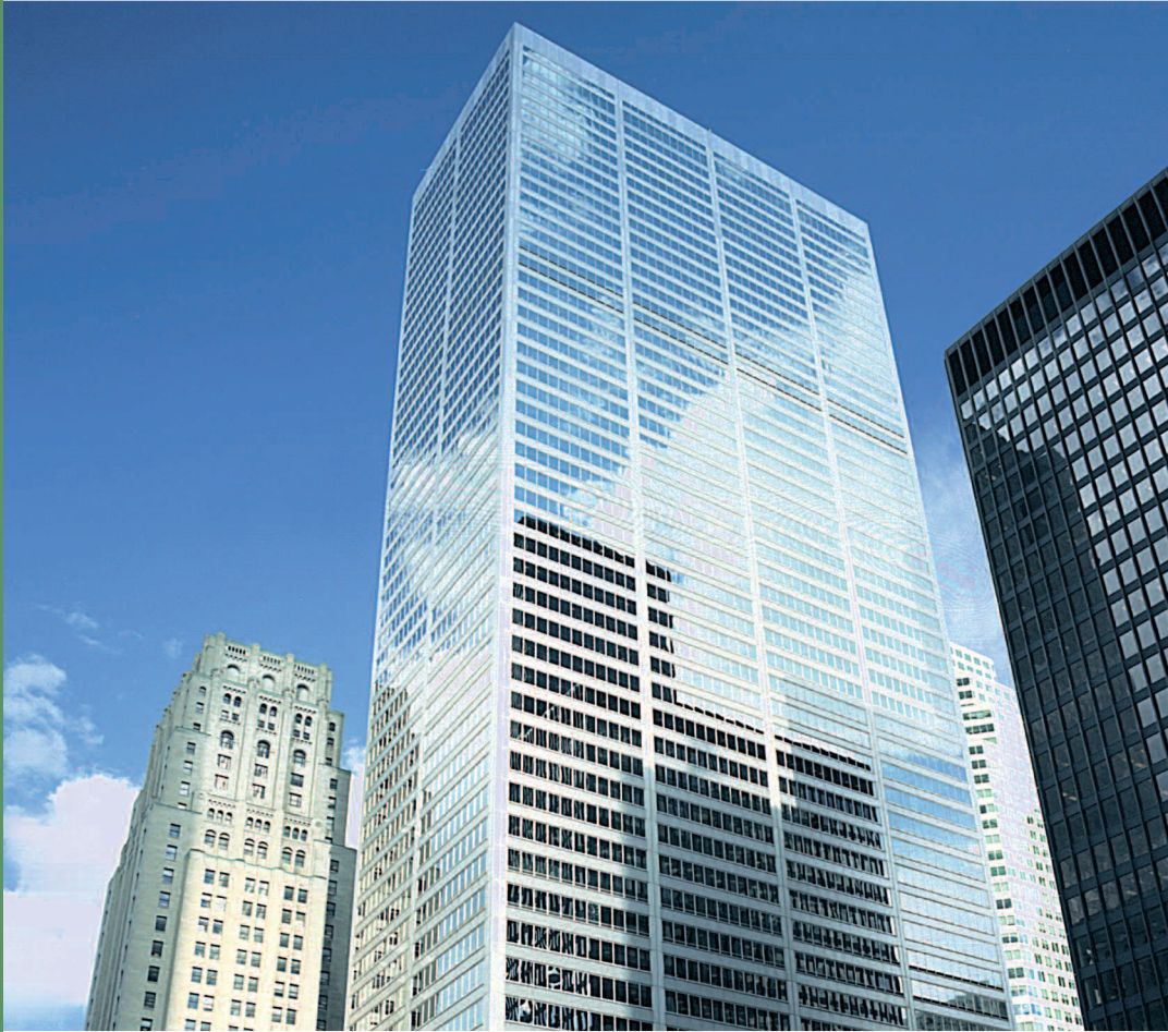
COMMERCE COURT, IN TORONTO, IS ONE OF CANADA’S PREMIER MIXED-USE COMPLEXES AND HAS ADOPTED POLICIES THAT HAVE SIGNIFICANTLY REDUCED ENERGY CONSUMPTION AND CARBON DIOXIDE EMISSIONS.
