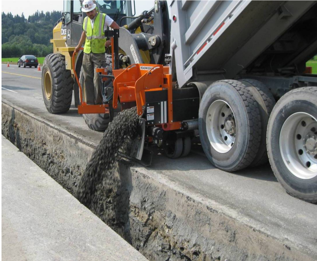
Figure 3-4: Kent Black Diamond Phase II Project, 16-Inch Diameter Supply Pipeline, In-Service 2009
