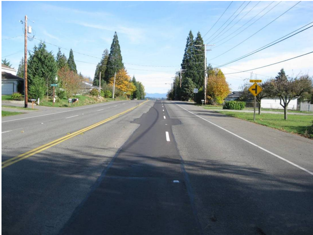
Figure 3-2: Kent Black Diamond Phase II Project, 16-Inch Diameter Supply Pipeline, In-Service October 2009
