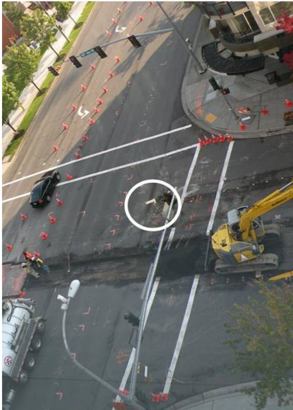
Figure 3-7: Bellevue Lake Hills 12- and 16-Inch-Diameter Supply Pipeline, In-Service 2009
