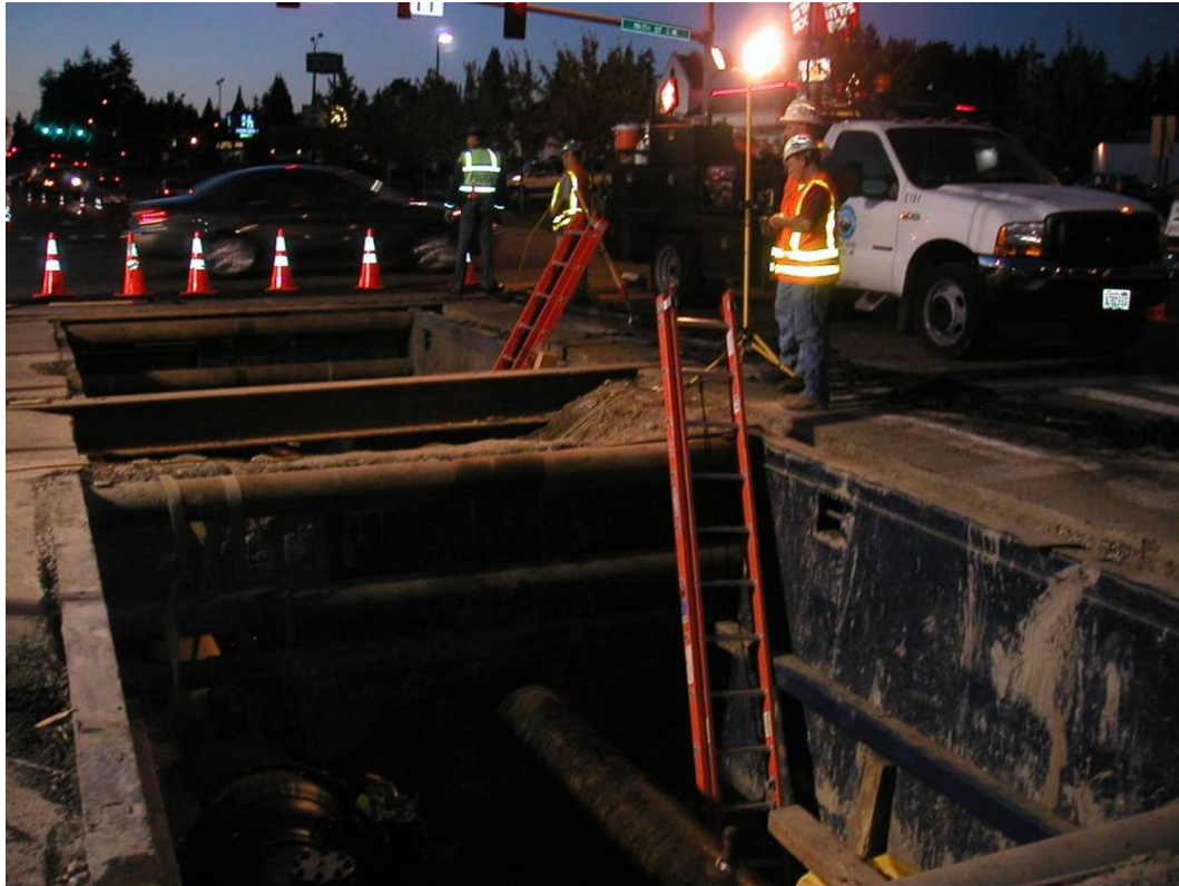
Figure 3-8: Lynnwood Valve Replacement, In-Service 2007
