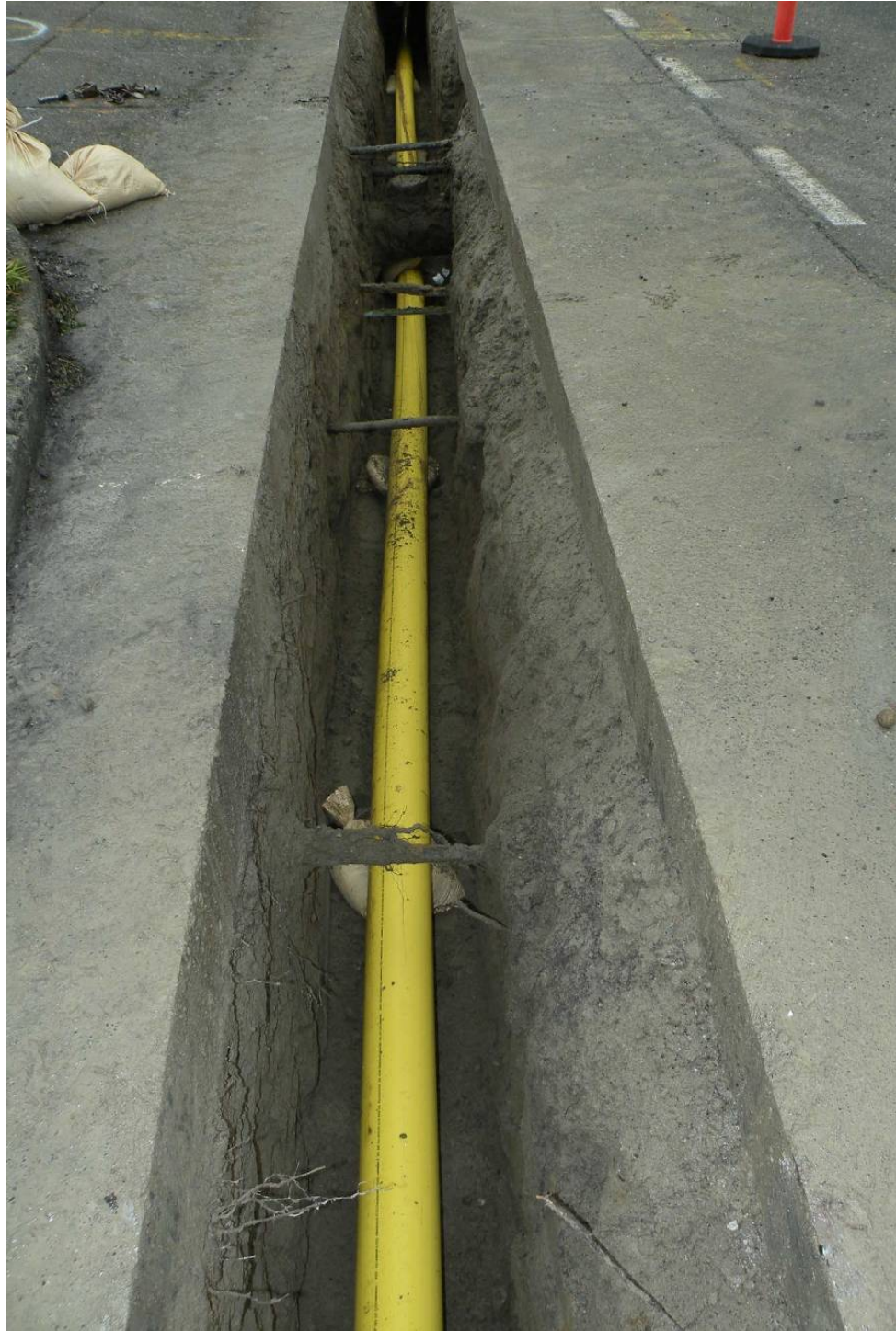
Figure 3-5: 6501 Beacon Ave S, 6-Inch Bare Steel Main Replacement, In-Service Expected 2010
