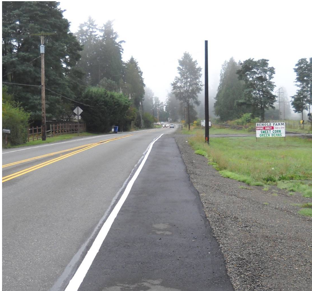
Figure 3-1: Orting Phase I Project, 8-Inch Diameter Supply Pipeline, In-Service 2007
