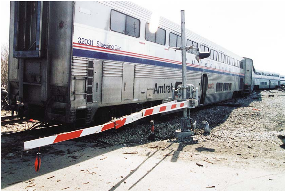
Figure 8. West (approach) crossing gate.
