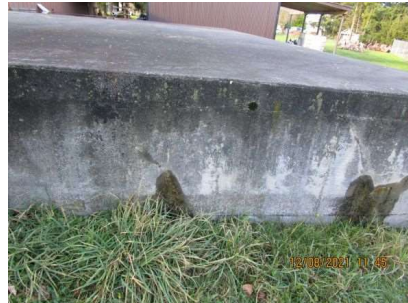
East Side Large Storage Tank
