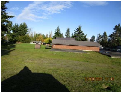
Water Facilities Site
