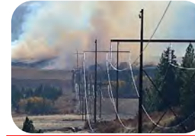
Operations & Emergency Response
