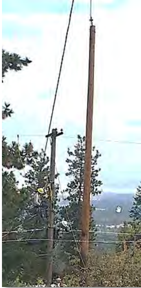
New pole being set with a crane
