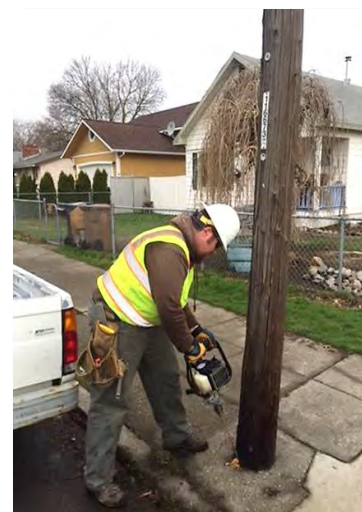
Avista Pole Inspection
