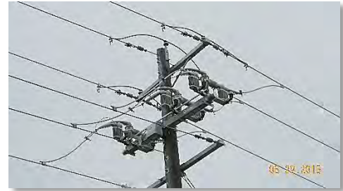
Above: Spokane Smart Grid Switching Device
