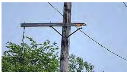
Above: Fire damaged pole Below: Broken crossarm
