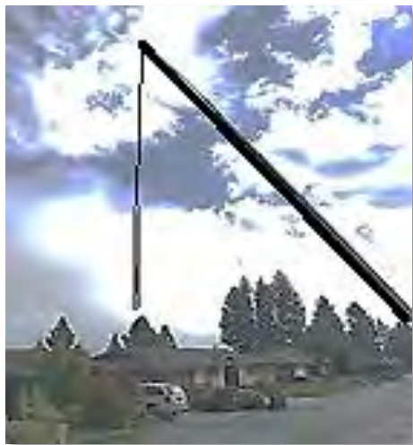
Above: Setting a pole in a backyard with a crane due to accessibility issues Below: Stuck in the mud
