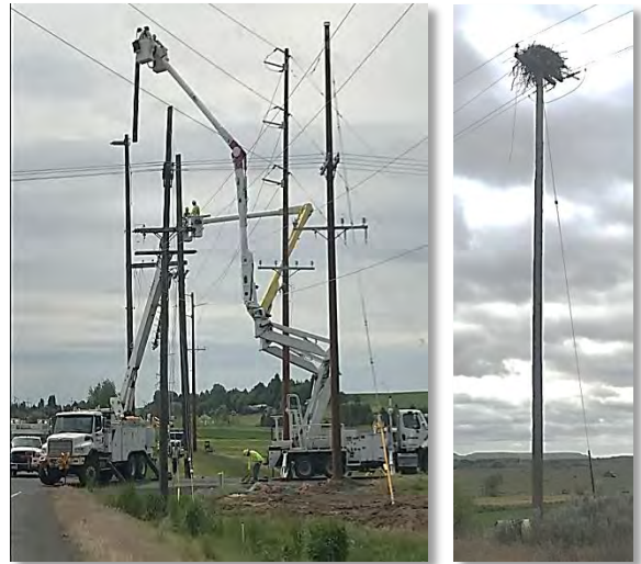
Left: moving poles and lines for a county road project
