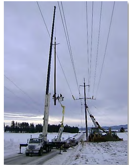
Transmission line repair in Coeur d'Alene District
