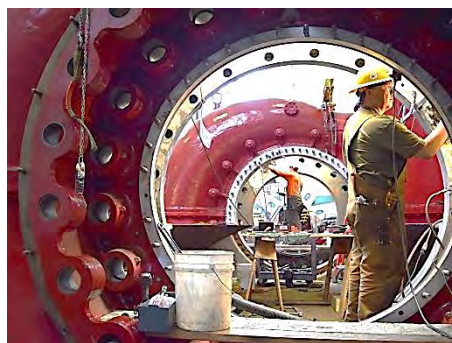
Maintaining a hydro unit
