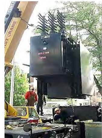
Placing a Pad Mount Transformer
