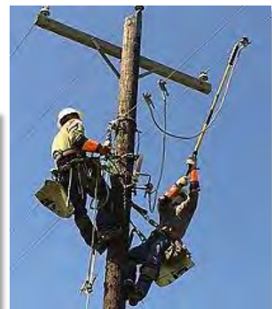
Using a “hot stick” to work on energized lines
