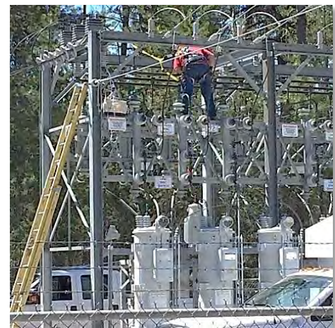
Working on a substation issue
