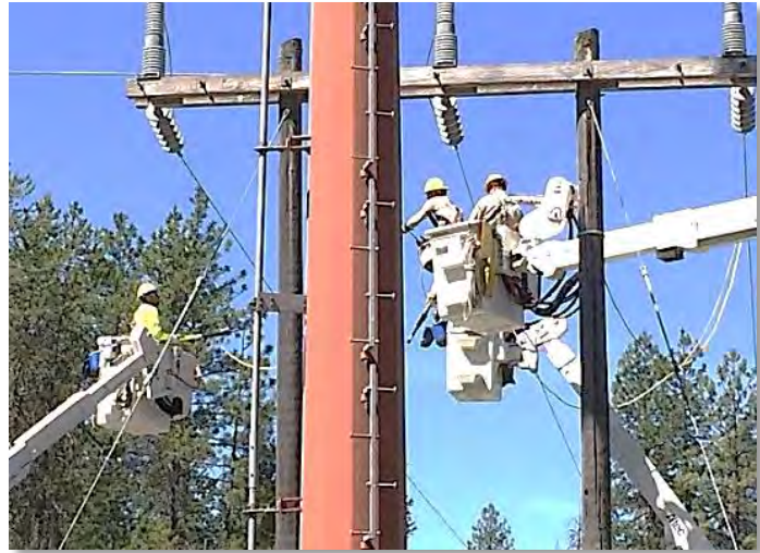
Deer Park Crew repairing transmission
