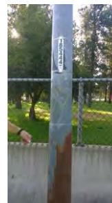
Figure 24: Pole Rusted
