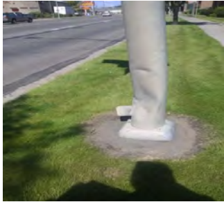
Figure 19: Pole Damage
