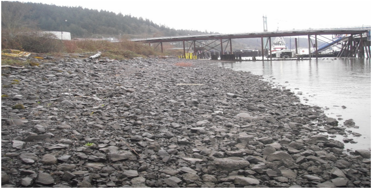
Photo 3 Conditions Immediately Downriver of Cap Area Looking Downriver (3/28/2023)
