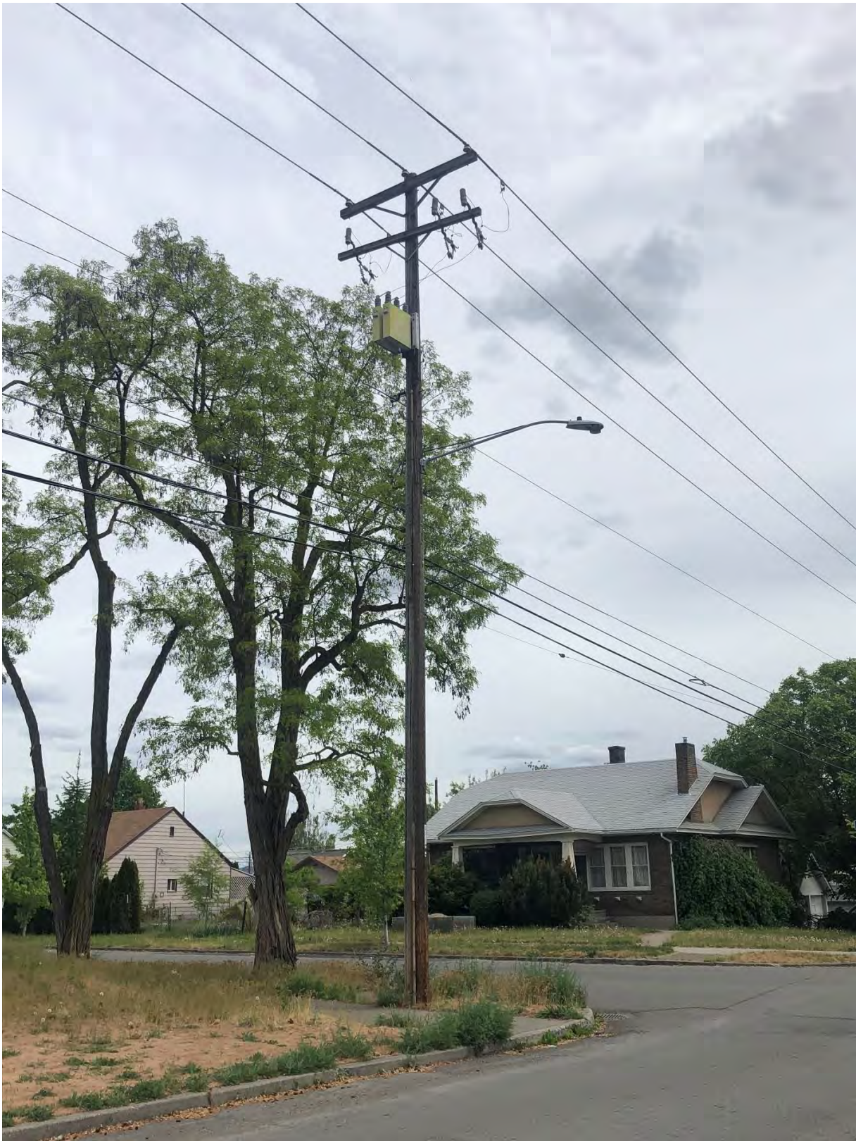
Figure 23. 600 kVAR 3-Bushing Style Capacitor Bank at Pole #084410
