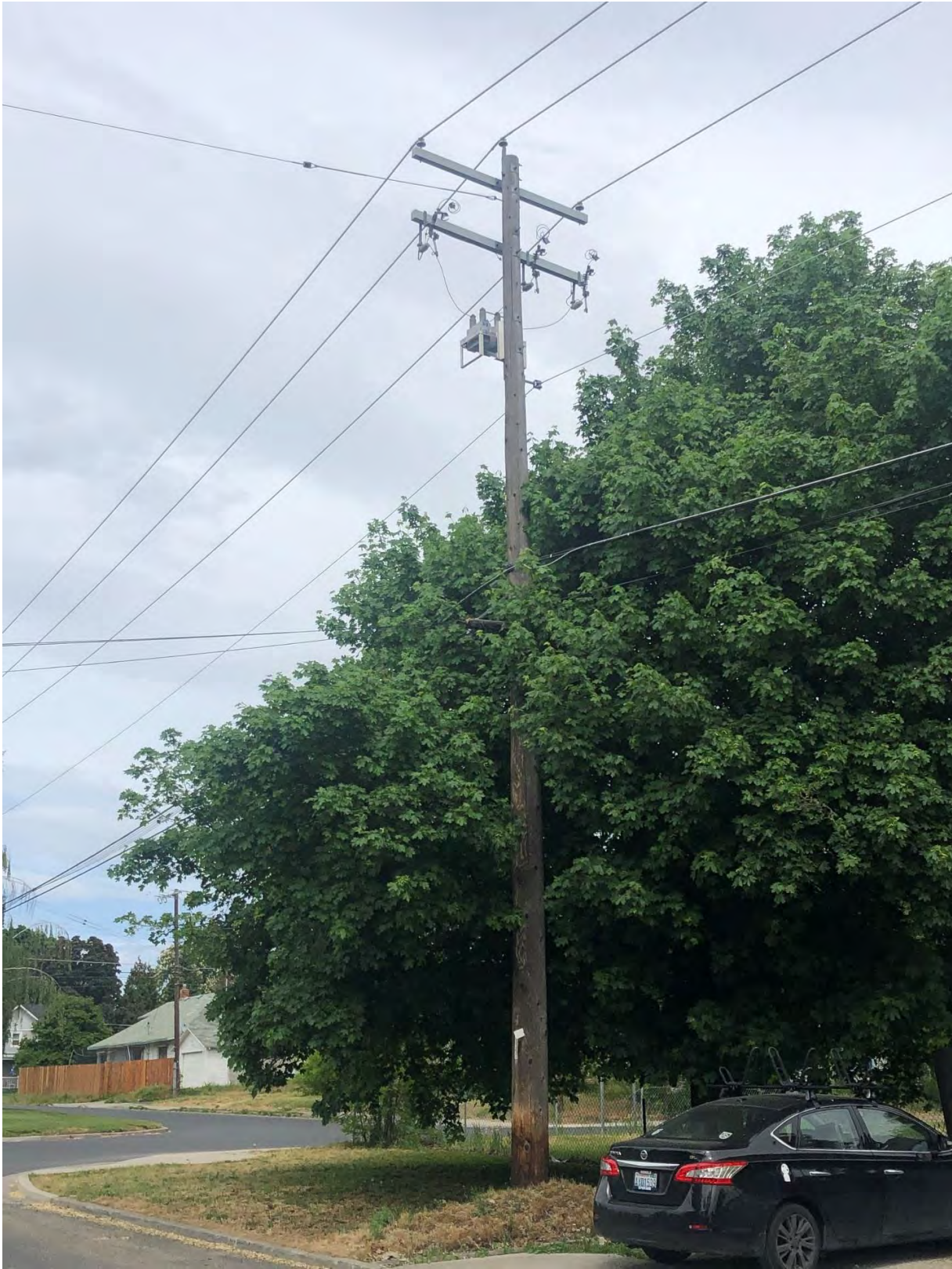
Figure 24. 600 kVAR 2-Bushing Style Capacitor Bank at Pole #303125
