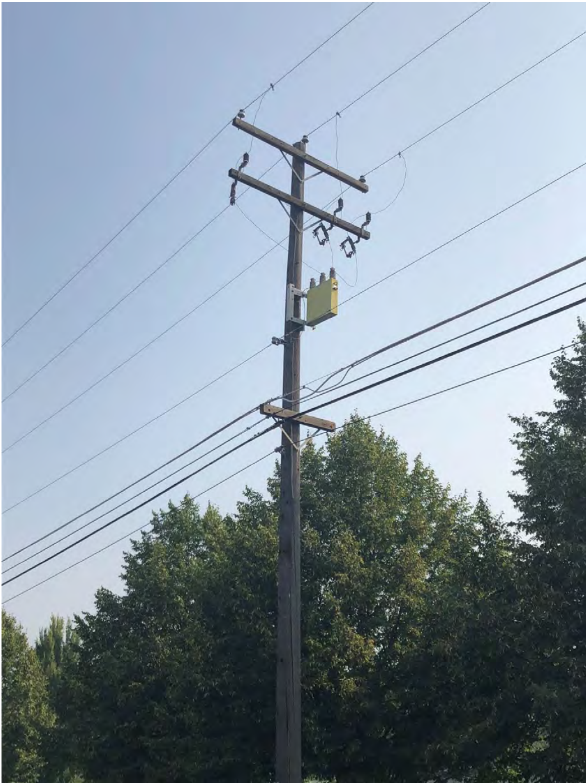
Figure 27. Existing 300 kVAR fixed, 3-bushing Style Capacitor Bank on SIP 12F4
