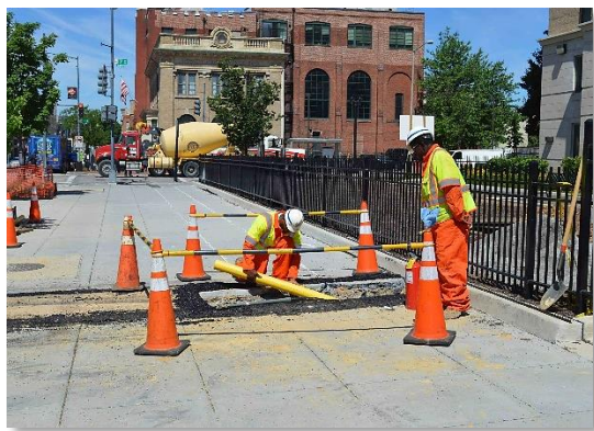
Natural Gas Pipeline Repair in Downtown Spokane
