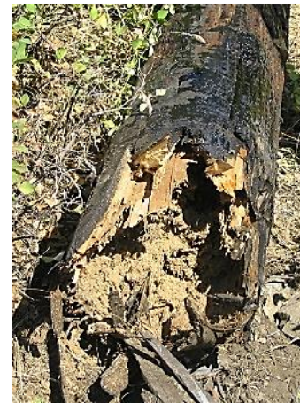
Pole rot causes a failure
