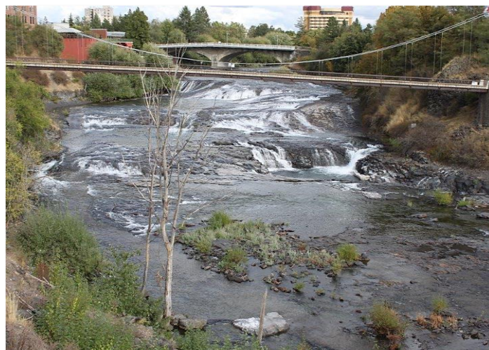
The North Channel of the Spokane River after Avista constructed weirs (small dams) in the river channel which were so cleverly designed that the approximately 170 cfs flowing in the river in this photo has the same appearance as 1500-1600 cfs did prior to the project completion. These weirs are indistinguishable to the public, as they were color and texture matched to blend in with the surrounding basalt channel.
