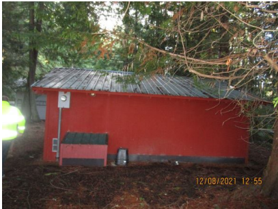
Pressure Tank Building
