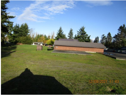
Water Facilities Site
