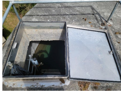
Tank 3 hatch & gasket
