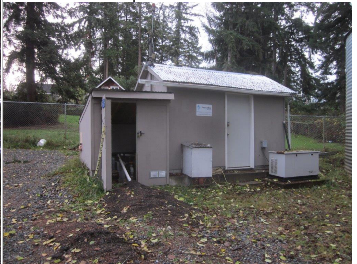
Pump house / well house
