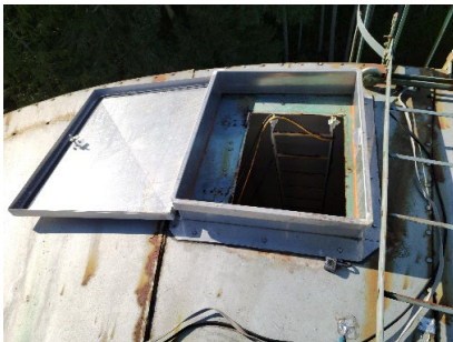
Tank 2 hatch & gasket
