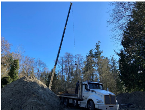
(Above) Construction is underway for the new reservoir
