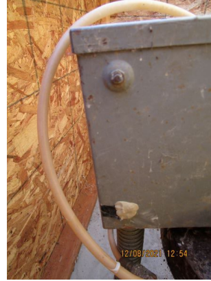
Well 2 – Junction Box Hole Filled
