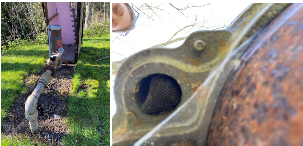
(L) Well #4 (R) Screened vent on Well #4 – screen bubbled but fully intact
