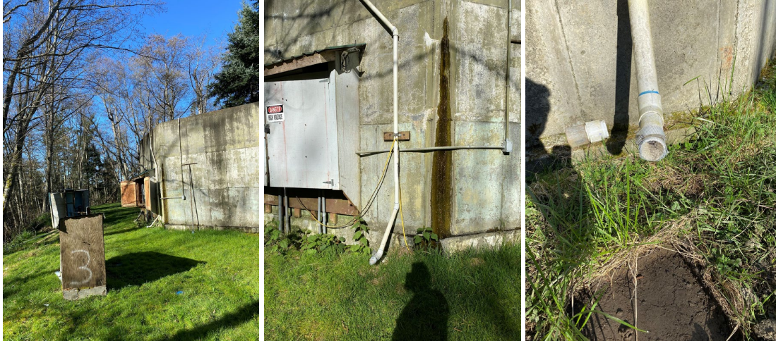
(L) Existing reservoirs with wells nearby (Center) Overflow for reservoir (R) Finer mesh needed for overflow screen
