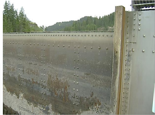
Above: Corrosion on Cabinet Gorge Spillgate #8 Left: Spillgates are subjected to a lot of different damaging factors, including river debris (Spillgate #6)
