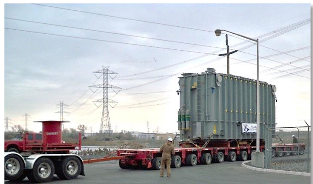
Coyote Springs 2 spare transformer being moved into place
