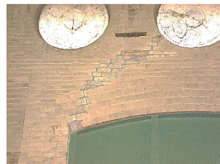
Repairs to a brick wall at Nine Mile
