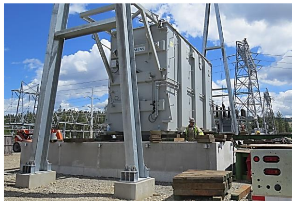
New Westside #1 230/115 kV transformer being placed
