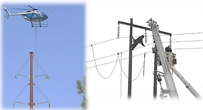
Placing conductor using a helicopter (left) and by hand (right)
