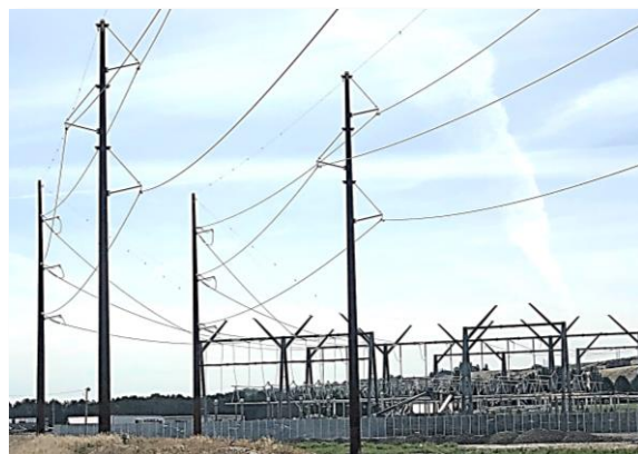
Saddle Mountain Substation under construction
