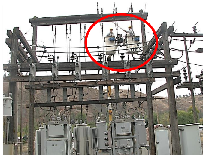
Work at the Kooskia Substation
