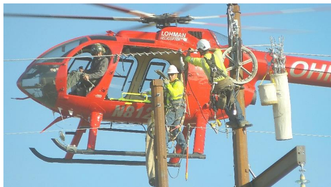
Working on the Benewah – Moscow 230 kV line
