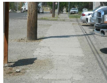
Avista parking area & sidewalk
