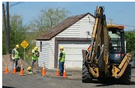
Avista gas crew uses a backhoe to dig up and repair a gas leak in Odessa
