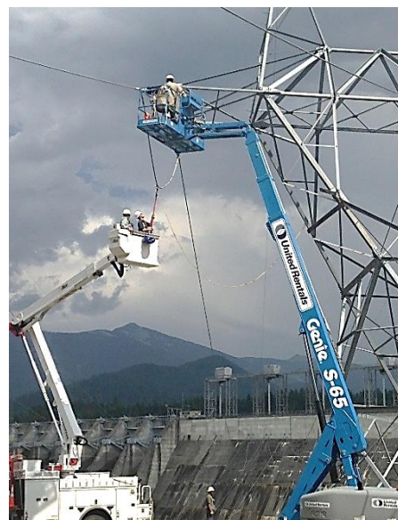
Bucket truck and Genie lift allow crews access to transmission tower at Noxon
