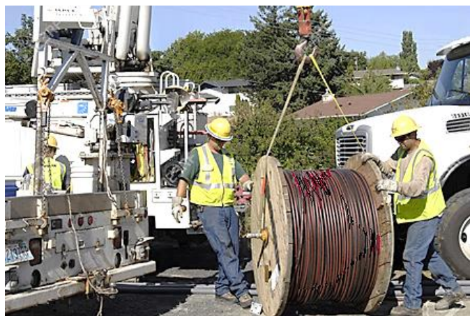
Avista service truck with a crane lifts a spool of cable
