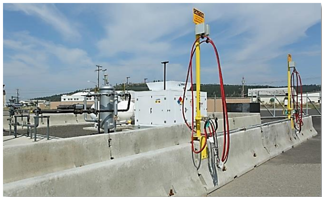
Compressed Natural Gas Fueling Station on Mission Campus
