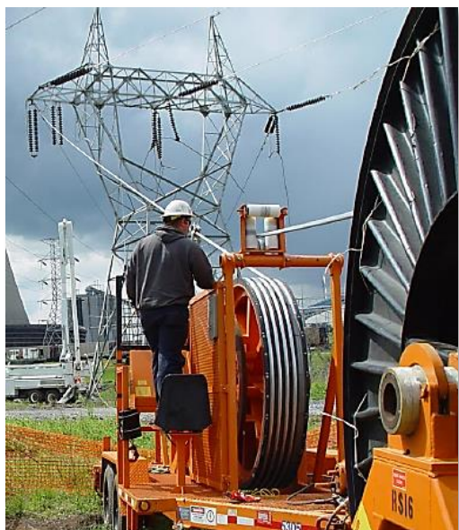
Puller-Tensioner stringing a high voltage transmission line
