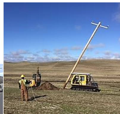
Using a small caterpillar to set a pole on Palouse farmland to minimize field damage
