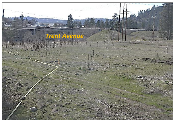
Site of new Irvin Substation in Spokane Valley
