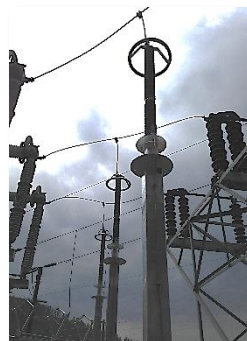
Lightning arresters at Lakeview Substation
