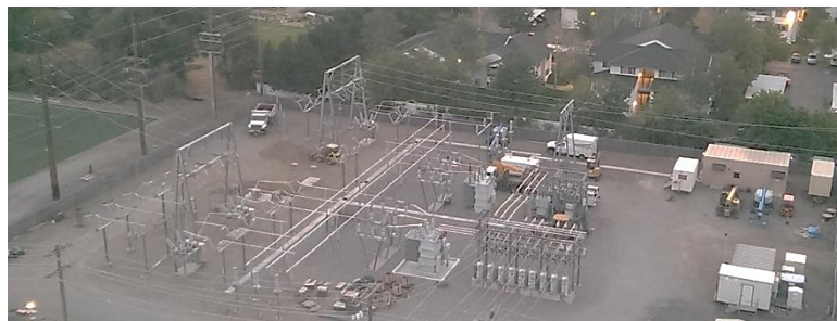
Building the Opportunity Substation in Spokane to manage customer growth
