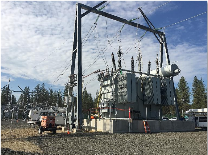
Installation of new autotransformer at Westside Sub
