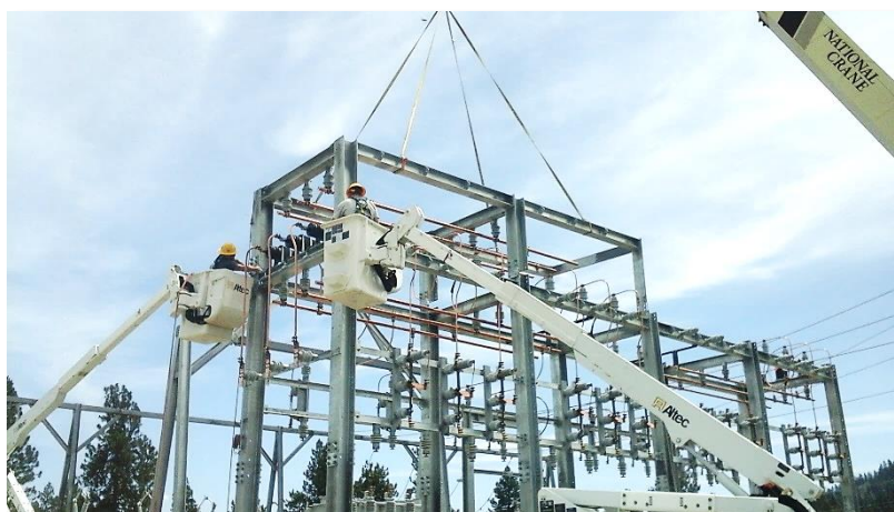
Work on the Ninth & Central Substation
