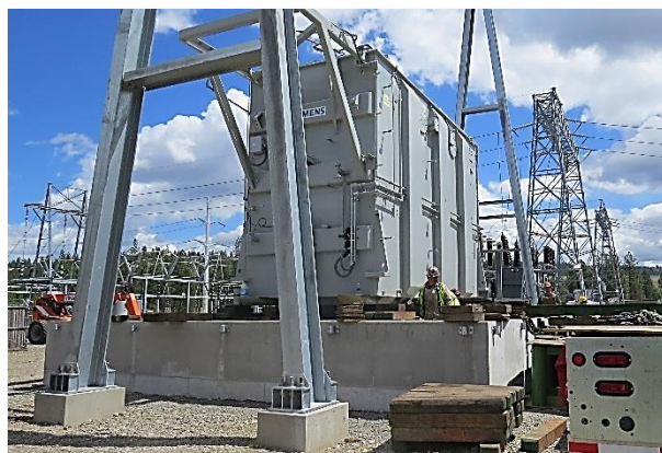
New Westside #1 230/115 kV transformer being put into place
