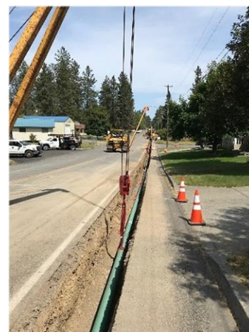
Gas Line Relocated for Road Work
