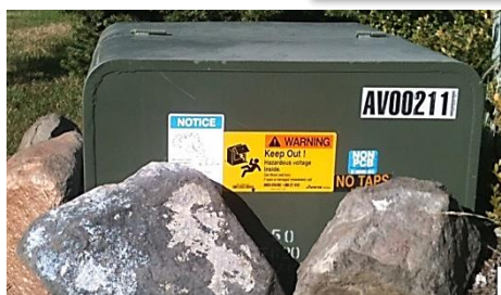
This program addresses required labeling such as the transformer decal above and access issues such as the boulders blocking access to the transformer on the left.
