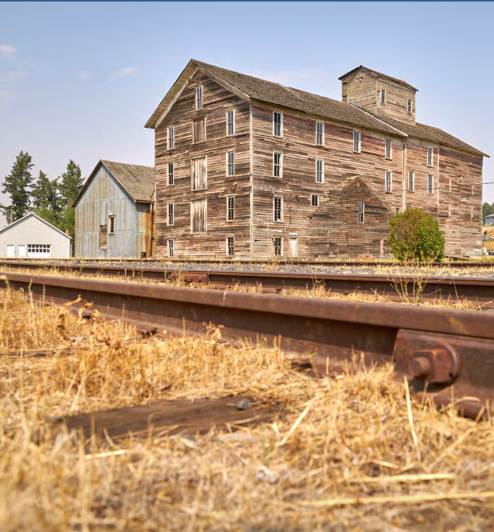
Historic Oakesdale Flour Mill, Oakesdale, Washington
