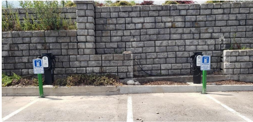
Figure 7: Workplace charging installation
