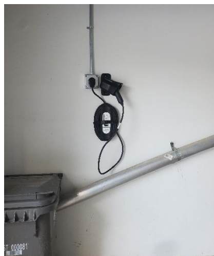
Figure 5: Residential charger installation
