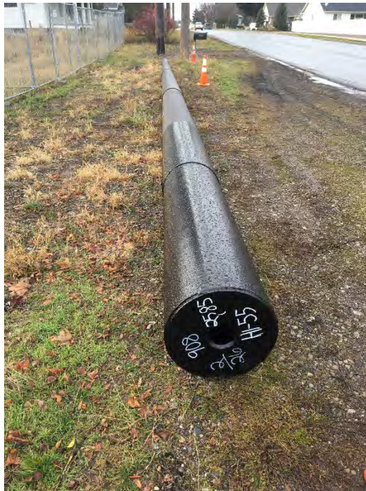
Efforts to Harden the distribution grid include the replacements of wood with steel poles. “High-Value Poles” in fire prone areas will be systematically replaced with steel to mitigate damage and outages during wildfire events.
