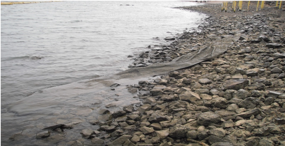
Photo 2 Organoclay Mat Material at the Downriver Extent of the Cap Area (12/22/2022)
