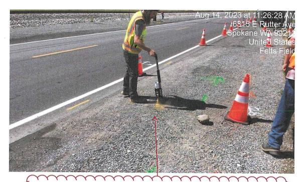
Locator marking live stub, 14 days after legally required date. live stub was only found because we found the abandoned line. not because Avista performed a legal locate that was accurate and timely. marker ball indicates end of live gas. EOM "end of main painted correctly after 14 days of legal dig
