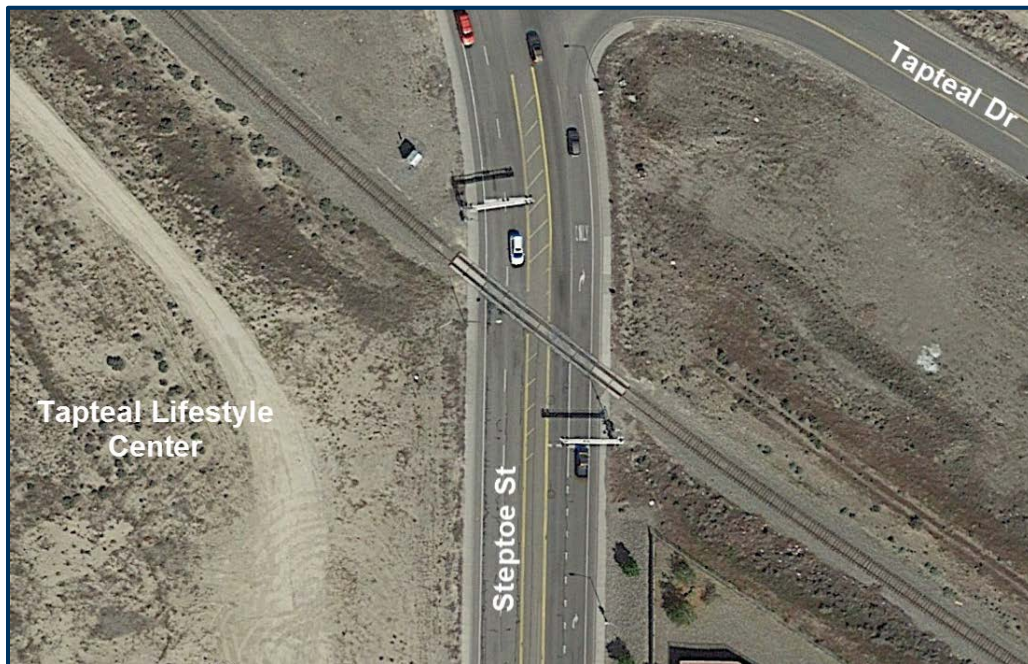
Photo 3 – Steptoe Street Grade Crossing
