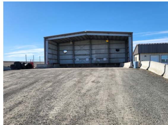
Figure 5-3. Ritzville Transfer Station
